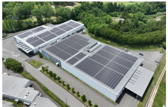
Hosorogi Facility, buildings 8/9
